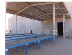
The John Campbell Miles Drill Core Storage Facility core viewing area
