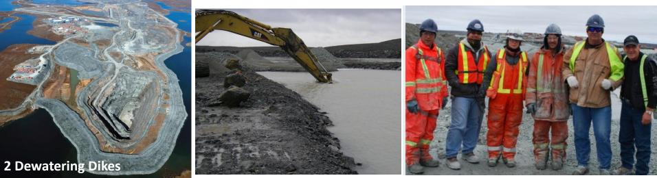
Length 3 km Max water depth : 8.5 m Max depth to bedrock : 22 m
